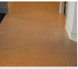
"Movement Joints – Vertical and Horizontal – EJ171" (page 78-80 in the 2009 version). This section gives a tremendous amount of information. It recommends movement joint placement every 20 to 25 feet in each direction for interior dry installations not exposed to sunlight and placement of movement joints every 8 to 12 feet in each direction for exteriors or interior sexposed to direct sunlight or moisture.
